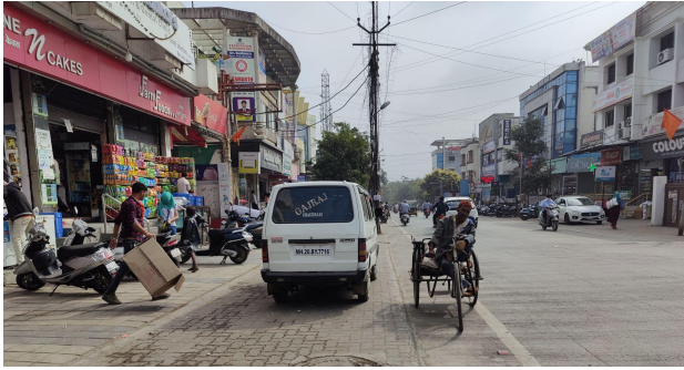
Image 12: Newly constructed road - At grade footpath facilitating parking upto property line.
