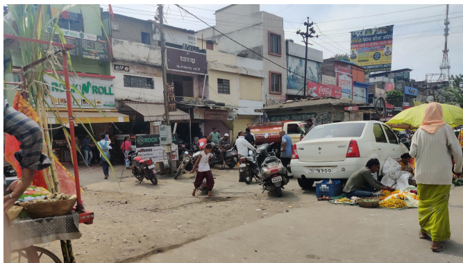
Image 15: Unpaved footpath space pushing pedestrians on carriageway
